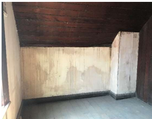
Figure 62 - Image describing the stained timber ceiling lining boards and the water damage to the side (southern) wall.
