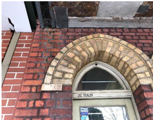
Figure 36 - Detail of the pointed brick arch and highlight window over the shop entry door.
