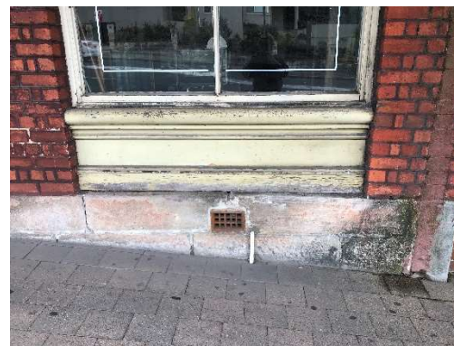
Figure 39 - Sandstone basecourse with timber bull nosed sill and mouldings and stall board. The terracotta vent appears to have been added later.
