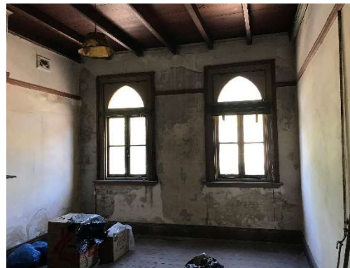
Figure 51 - Interior view of the pointed arch head windows facing the Pacific Highway on the first floor. Note the ceiling structure, being the underside of the flooring to the second floor spaces.
