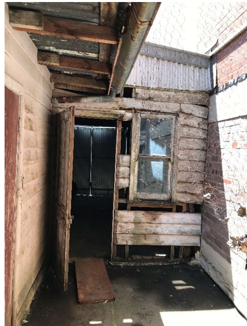
Figure 47 - A partial view of the rear shed construction. This weatherboard section appears earlier than later concrete and corrugated iron construction. Note the construction of the later commercial building to the right of the image.
